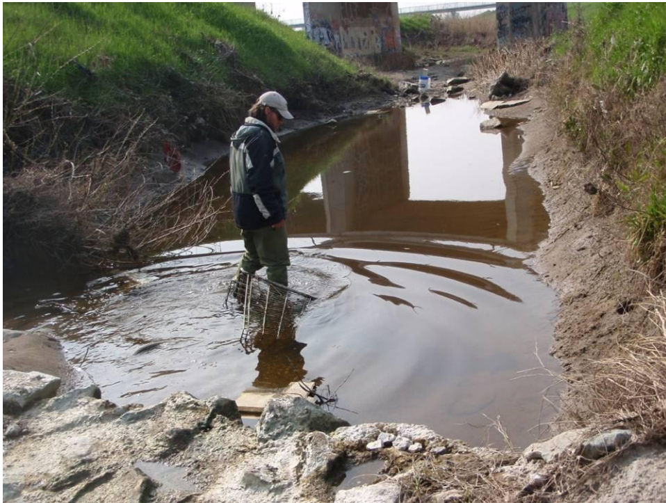
Figure 9. Feb. 18, 2010. Pool at the culvert downstream of the footbridge and RR bridge.
